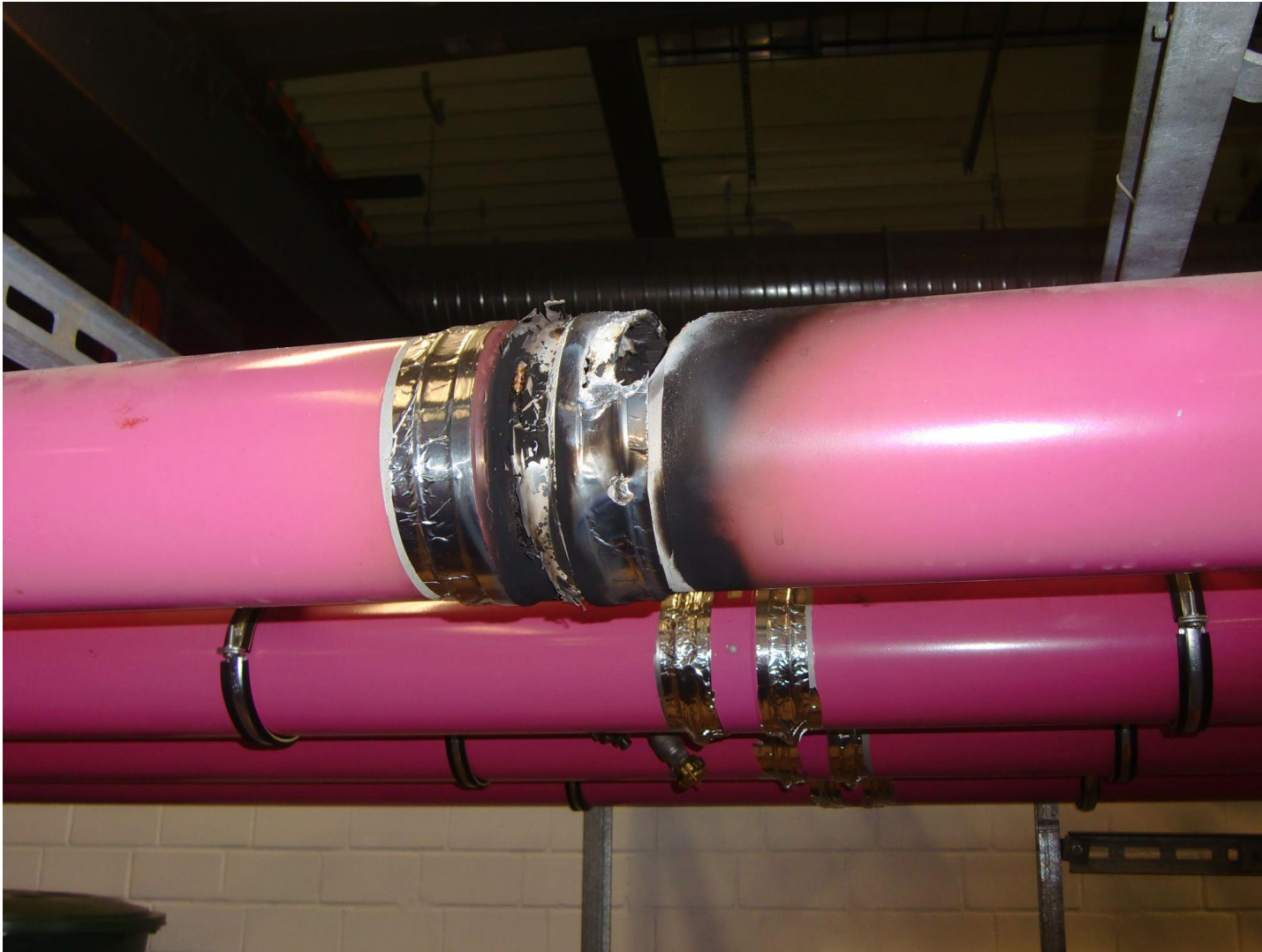
Burned coaxial power line
